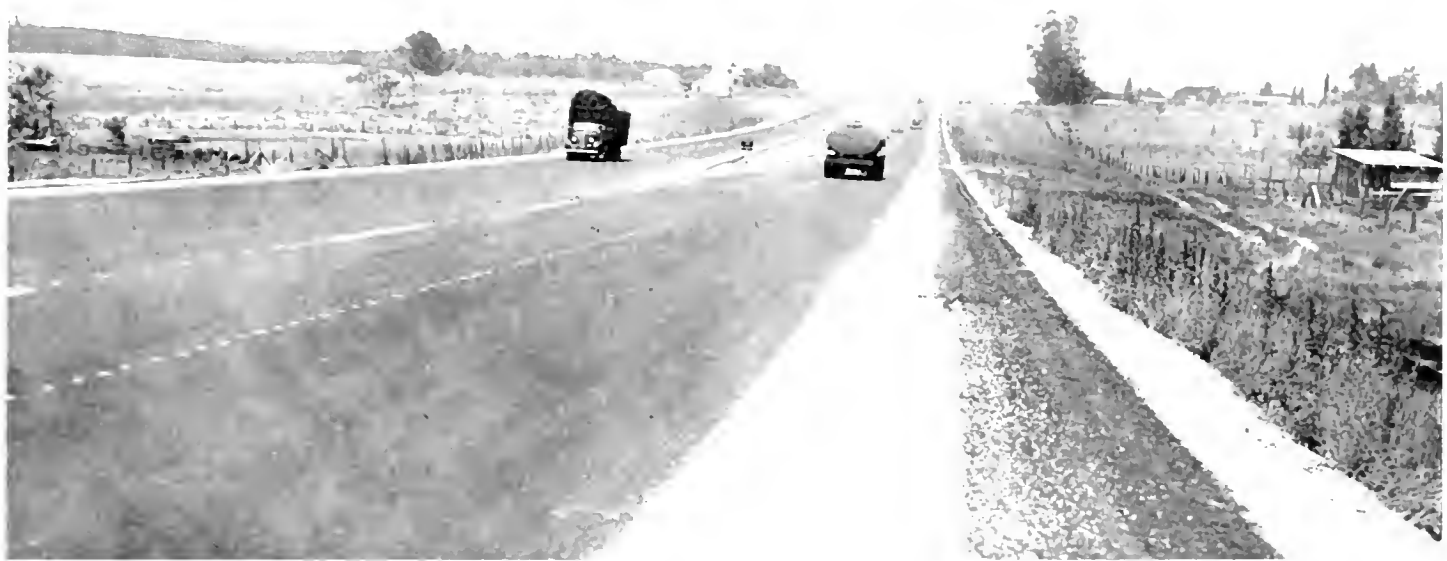
View showing transition section where divided highway merges into two-lane existing highway ahead at end of project
